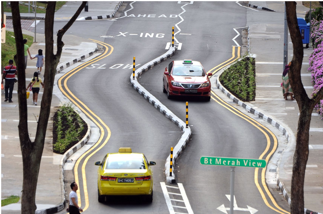
Figure 44: A chicane used in Singapore's Silver Zone (image from LTA) 62
