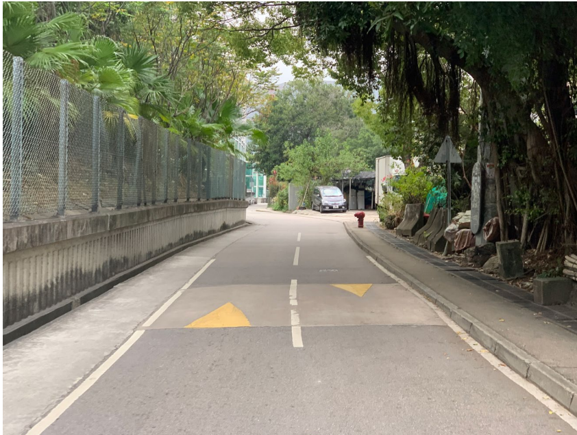
Figure 39: A speed hump installed on a village road in Tuen Mun
