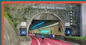
獅子山隧道 步行及單車通道 Second Lion Rock Tunnel Walking and Cycling Path
