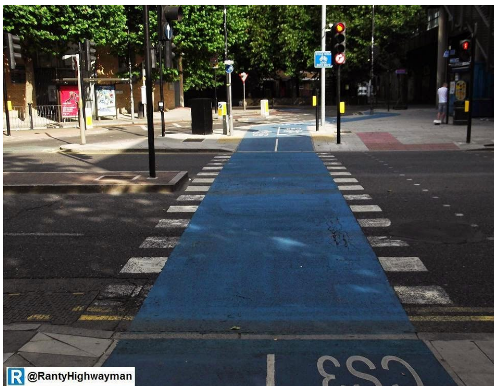
Example of a signalised parallel crossing for cycles seen in London's Cycle Superhighway 3 (credit: RantyHighwayman)
