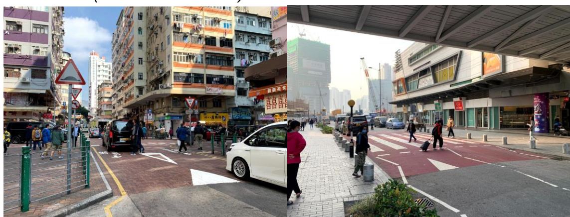
A raised table junction trialled in Shum Shui Po and a mid-link raised table zebra crossing trialled in Kai Tak
